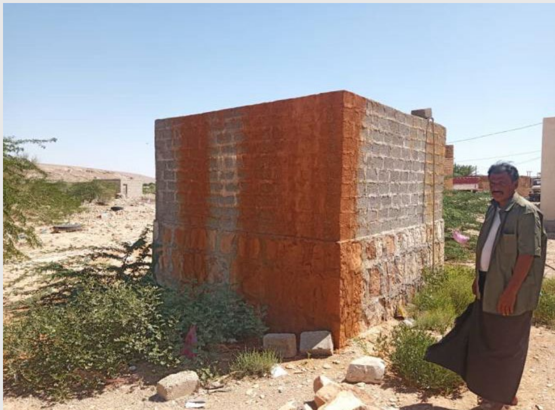
Figure 7: Water tank with iron residues
