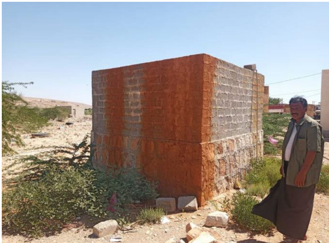
Figure 7: Water tank with iron residues
